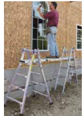
POSITION #4 Self-Supporting 2-Scaffold
